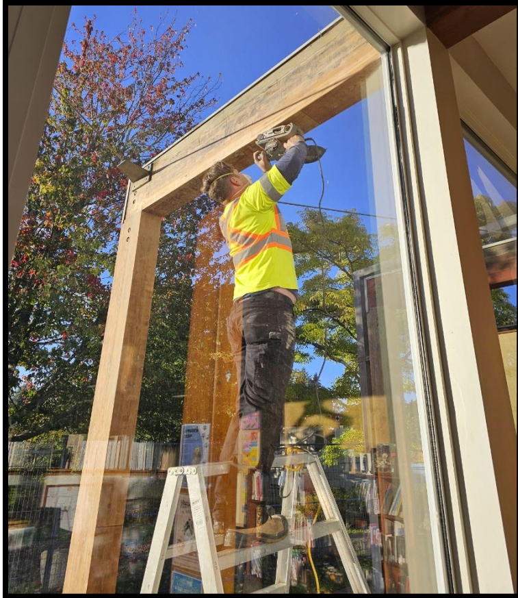
Sanding of all the beams back to a natural state
