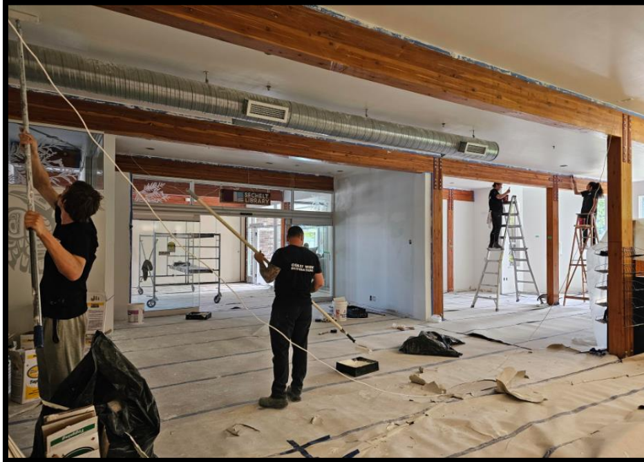
Coast wide team completing the painting of the ceiling and walls.
