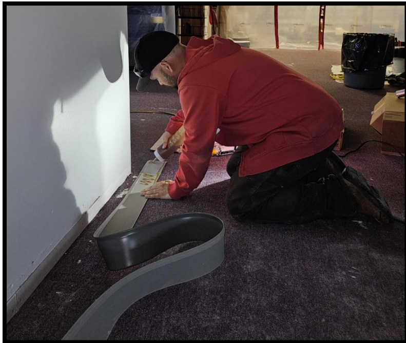
Paul, a local subcontractor, putting on the COVE baseboards
