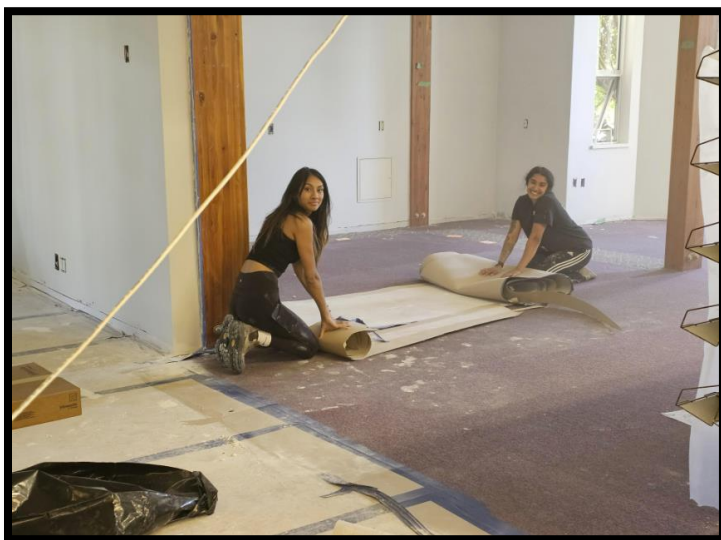
Thursday June 13 – Coast wide team picking up floor coverings
