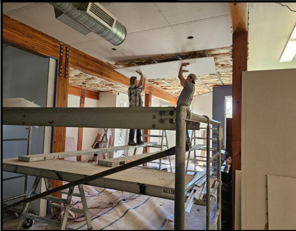
Left: Drywallers completing the ceiling
